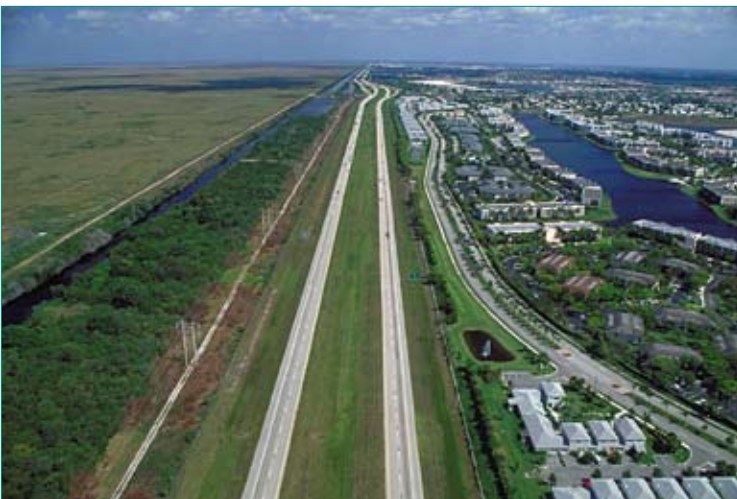
Human development encroaches on natural ecosystems, affecting the quality and quantity of water available to them. Here, a highway divides a development from a water conservation area in South Florida. Photo courtesy of the South Florida Water Management District.
