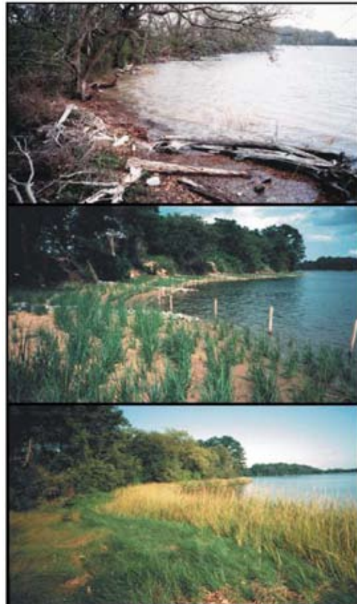
Planting vegetation offers an alternative for reducing erosion at some sites. Top photo shows a pre-project shoreline on Wye Island in Queen Anne's County, Maryland. Marsh grass was planted on sand fill and short, stone groins were placed. Middle photo is three months after installation. Bottom photo is six years after installation. Source: Hardaway and Byrne (1999).
