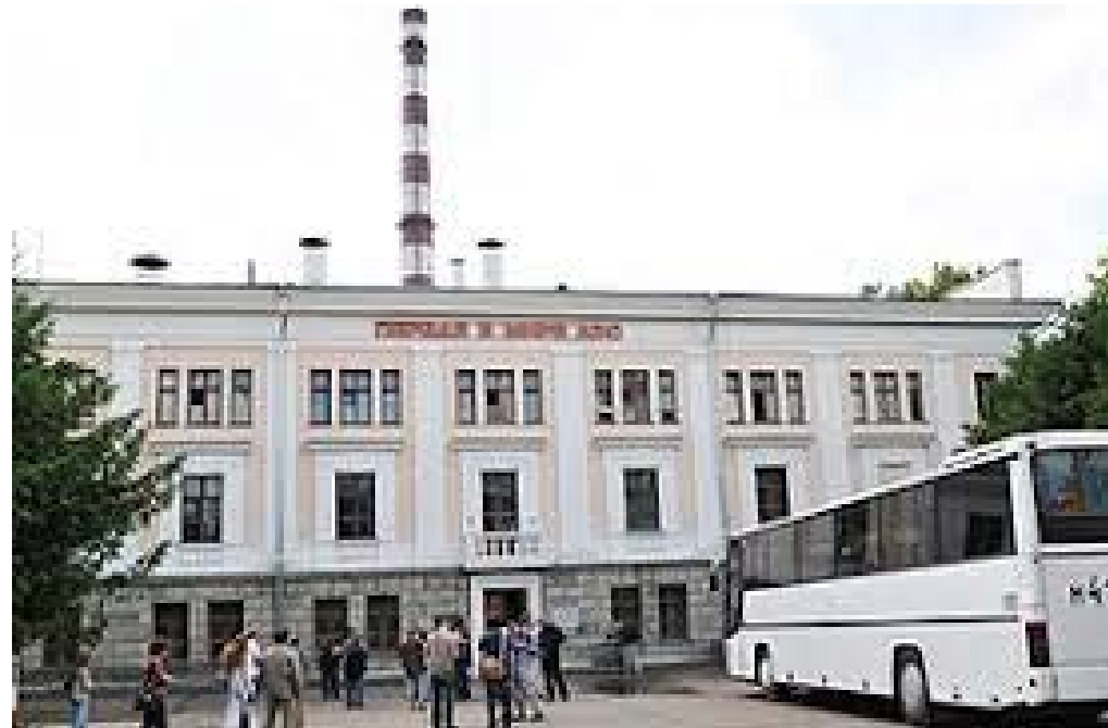
Obninsk Nuclear Power Plant
